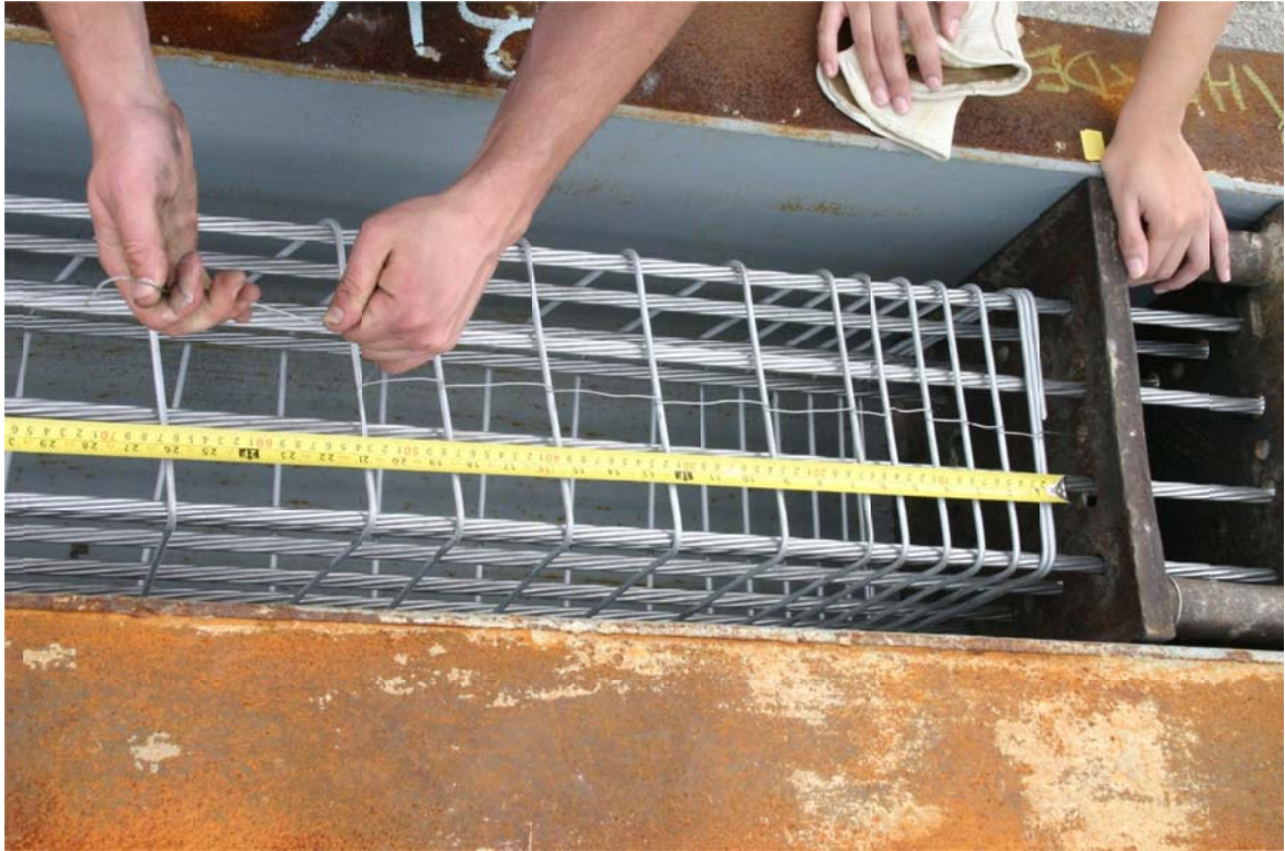
Figure 5.11 Spirals restrained by continuous stainless steel tie wire.
