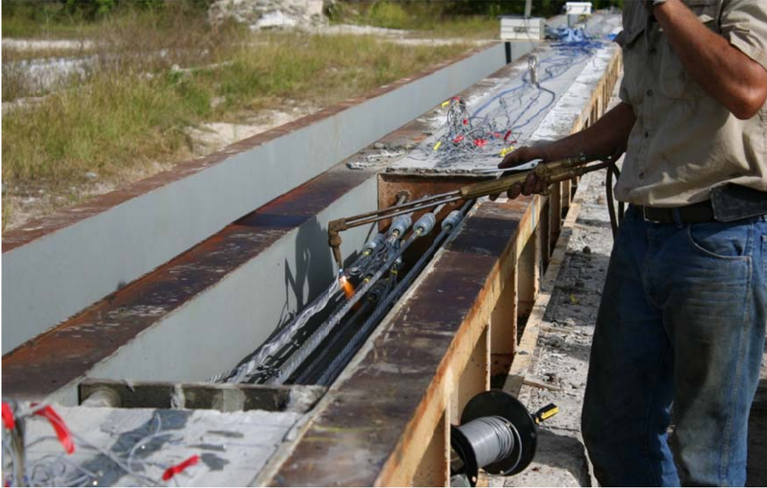
Figure 5.26 De-tensioning performed by cutting strands with a torch.
